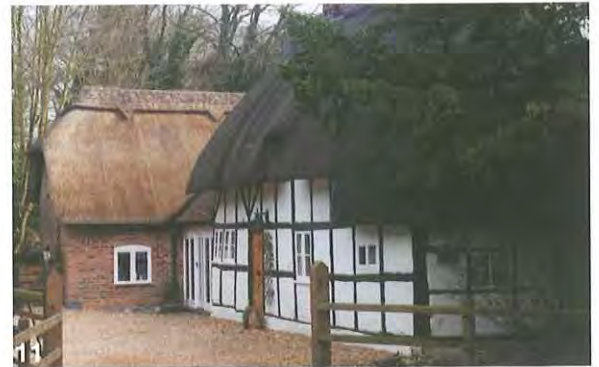
10. Northbrook Arms and 22-31 East Stratton Lane, East Stratton
